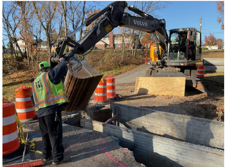
NE 10th St – Storm Water Improvements
