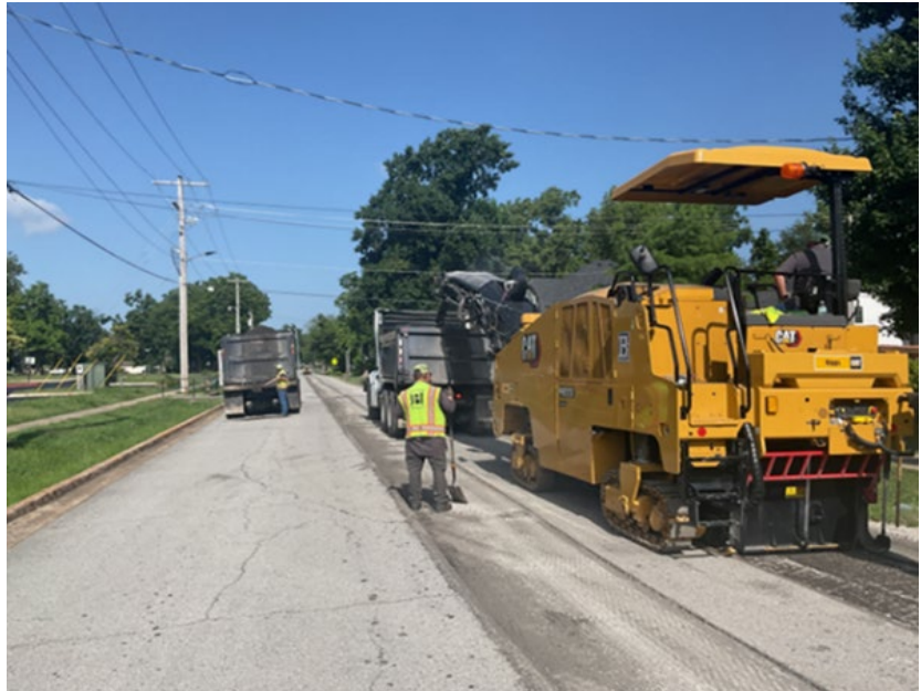
2NW 3rd St – Asphalt Cold Planning
