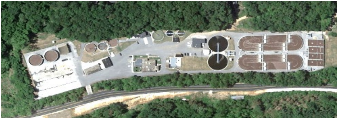
Bentonville Wastewater Resource Recovery Department located on 1901 NE A St,
