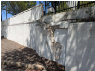
E Chicago/S Grove retaining wall
