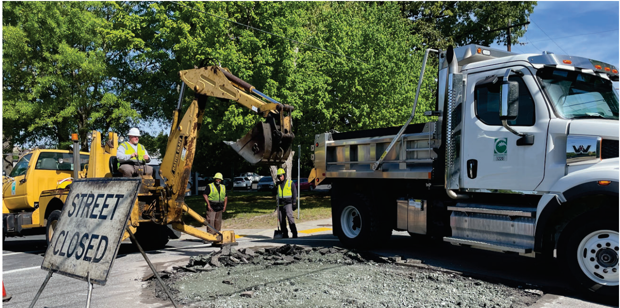
Greensboro Department of Transportation (GDOT) repairing street asphalt
