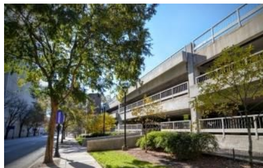
Raleigh Municipal Parking Deck
