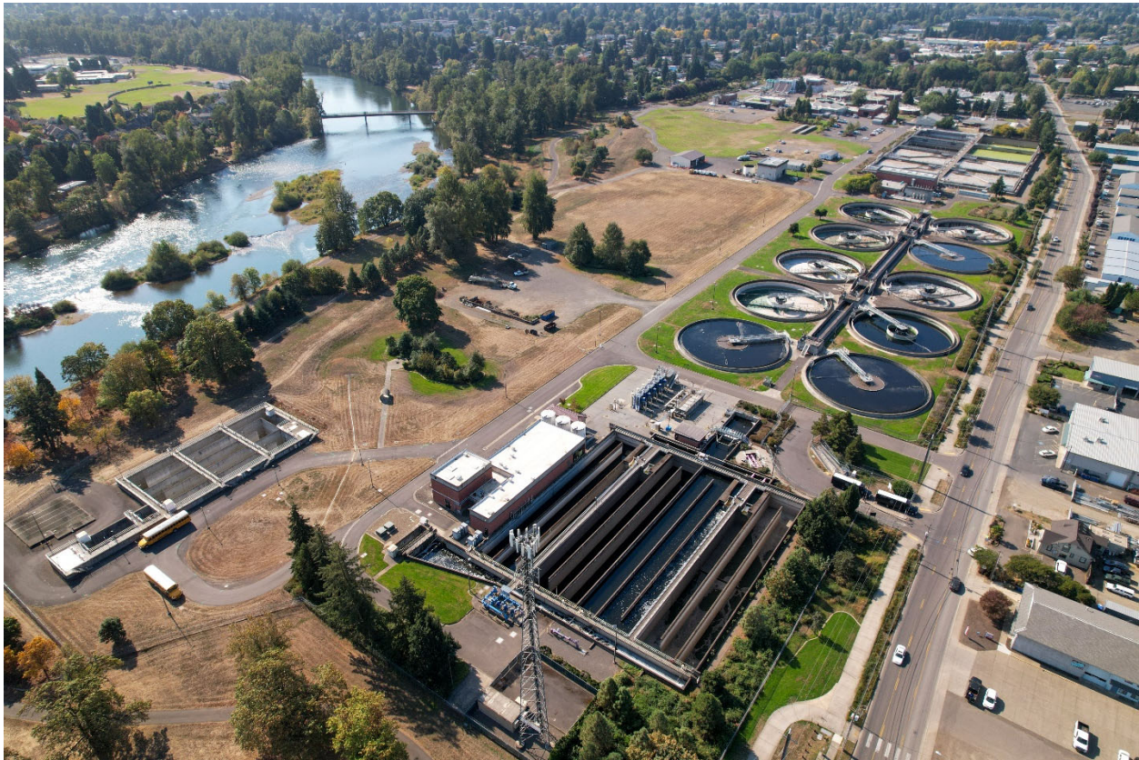
Regional Wastewater Treatment Plant (also known as the Water Pollution Control Facility)
