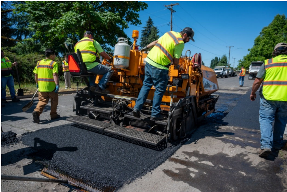
53 rd Place Surface Drainage
