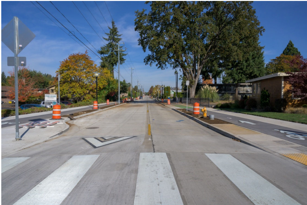
Mill Street Reconstruction, 2025
